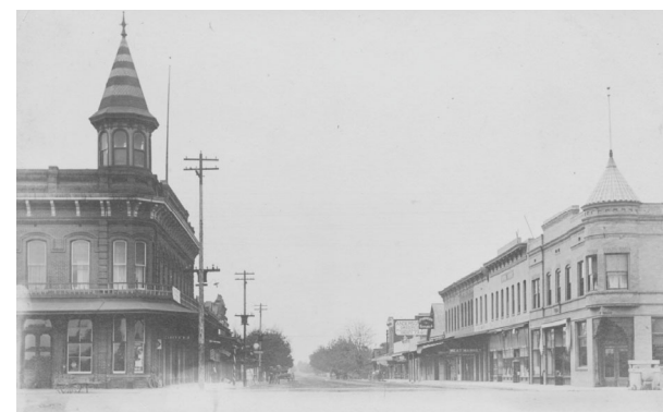
Main Street looking west from Railroad Avenue. Photo I11-005. Acc. #1993-015.
