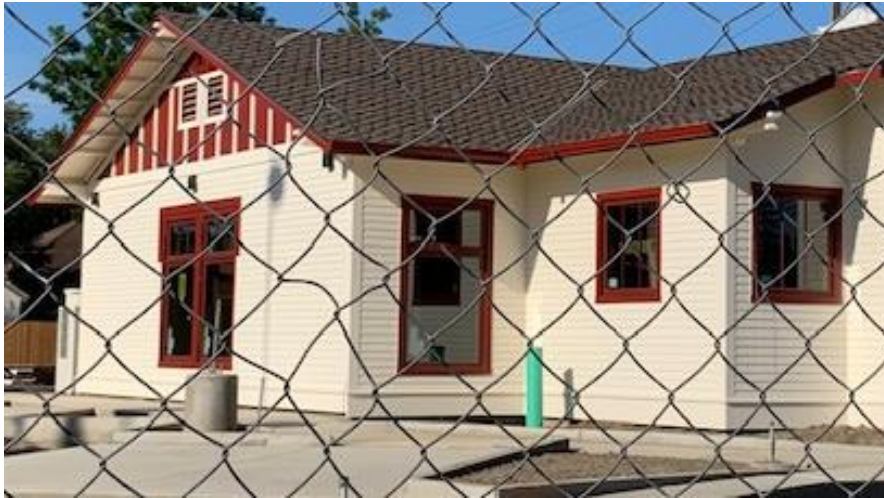
Exterior of the new Yolo Branch Library – recently painted!
