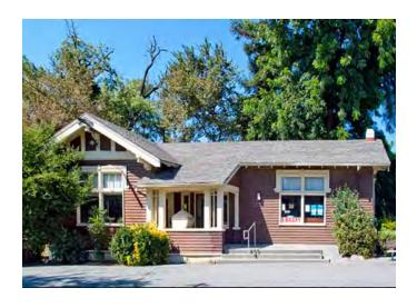
The current historic Carnegie building is 1,000 square feet, and is on the Yolo County Capital Project List 2015-2018 to be replaced. In 2013 dollars, there were \$188,278 in current deficiencies. In addition to priority code compliance with fire and life safety, there are structural (foundation), plumbing, electrical, roofing, interior, and exterior deferred maintenance concerns, as well as ADA compliance issues.
