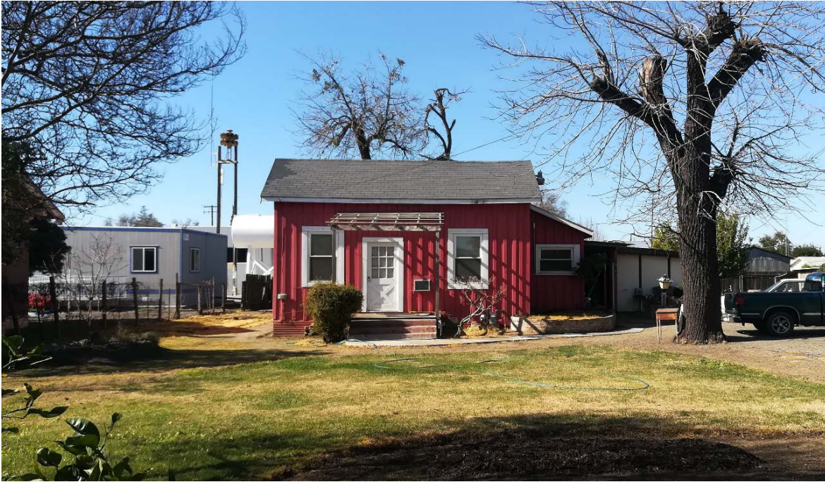
Figure 2-3 Site Photos (Residential Property at 14184 2 nd Street)
