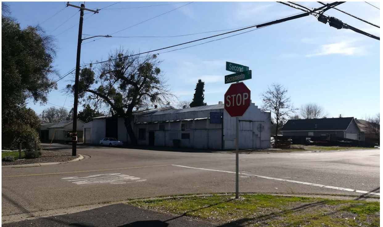
Figure 2-4. Top: View looking northwest to the existing Yolo Branch Library building. The Yolo Fire Station is located left of center in the photo. The temporary modular building was not yet installed at the site (photo date January 2017). Bottom: View from the Yolo Branch Library property looking southeast across the intersection of 2 nd Street and Sacramento Street (photo date February 2018).
